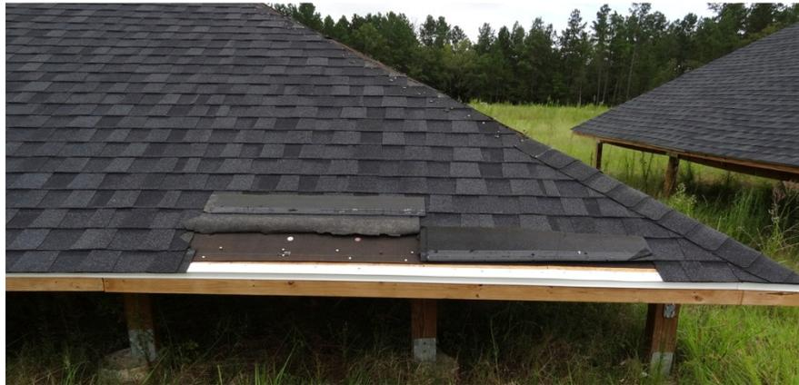
**Fig. 137. Pull-through eave starter strip shingles at fasteners causing cracking to the surface of first and second shingle courses (LAM-201 – Roof 6).**
