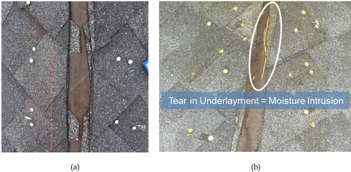
**Fig. 136. Underlayment wrapped over hip line: (a) likely water-resistant (LAM-201 – Roof 4) and (b) torn underlayment likely due to roof installers cutting field shingles at the hip line causing exposure of hip line to moisture intrusion (LAM-202 – Roof 6).**
