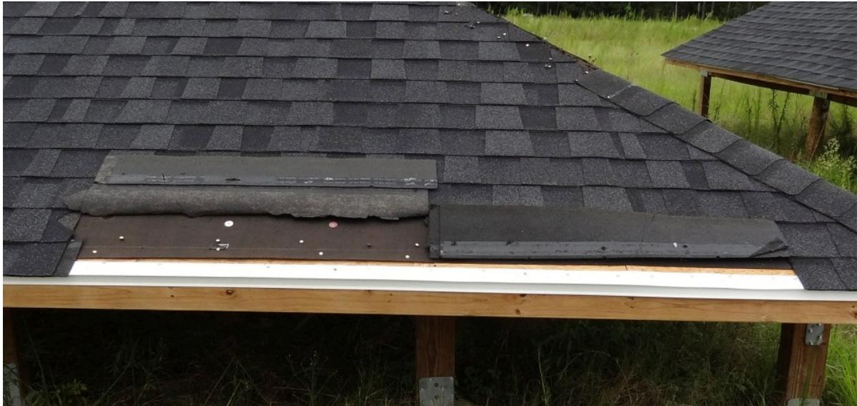
**Fig. 113. Pull-through of the starter strip around fasteners on LAM-201 – Roof 6. The fasteners were placed approximately 102 mm (4 in) from the butt edge of the starter strip.**
