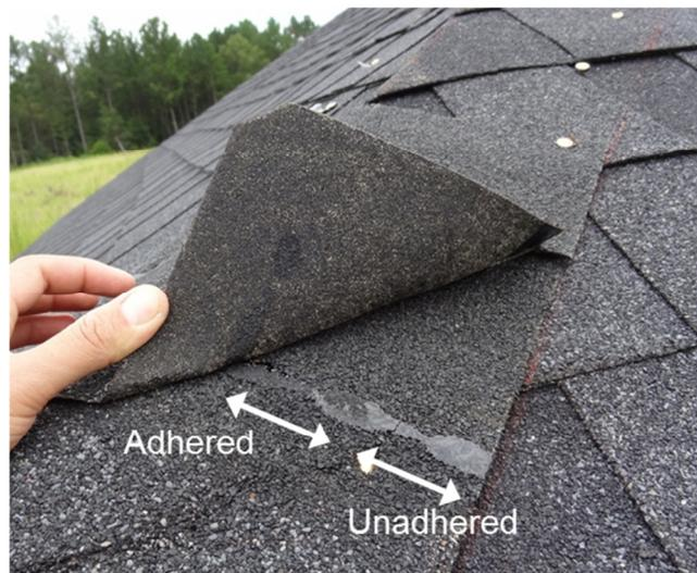
Fig. 131. Example of unsealed hip shingle on LAM-201 – Roof 5. The shingle was unadhered at the edge of the hip shingle and adhered closer to the center of the hip line. (Note: this photo was taken after wind testing.)
