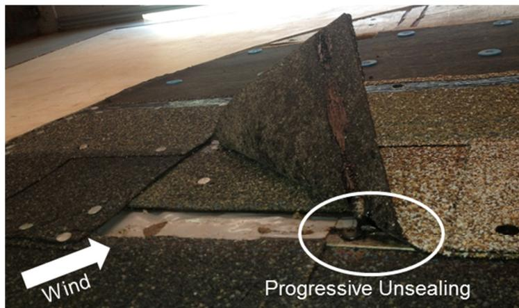
Fig. 88. Progressive unsealing observed on partially unsealed laminate shingle specimen.
