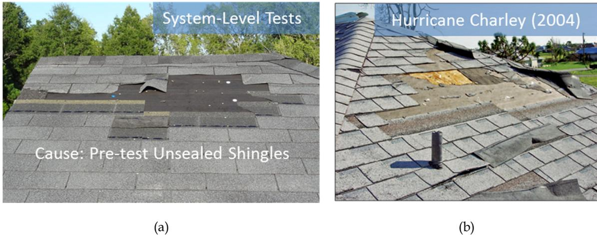
**Fig. 139. (a) Shingle blow off obtained from system-level performance test caused by pre-test non-bonded shingles and (b) blown off shingles observed by FEMA after Hurricane Charley [Photo from FEMA (2011)]**
