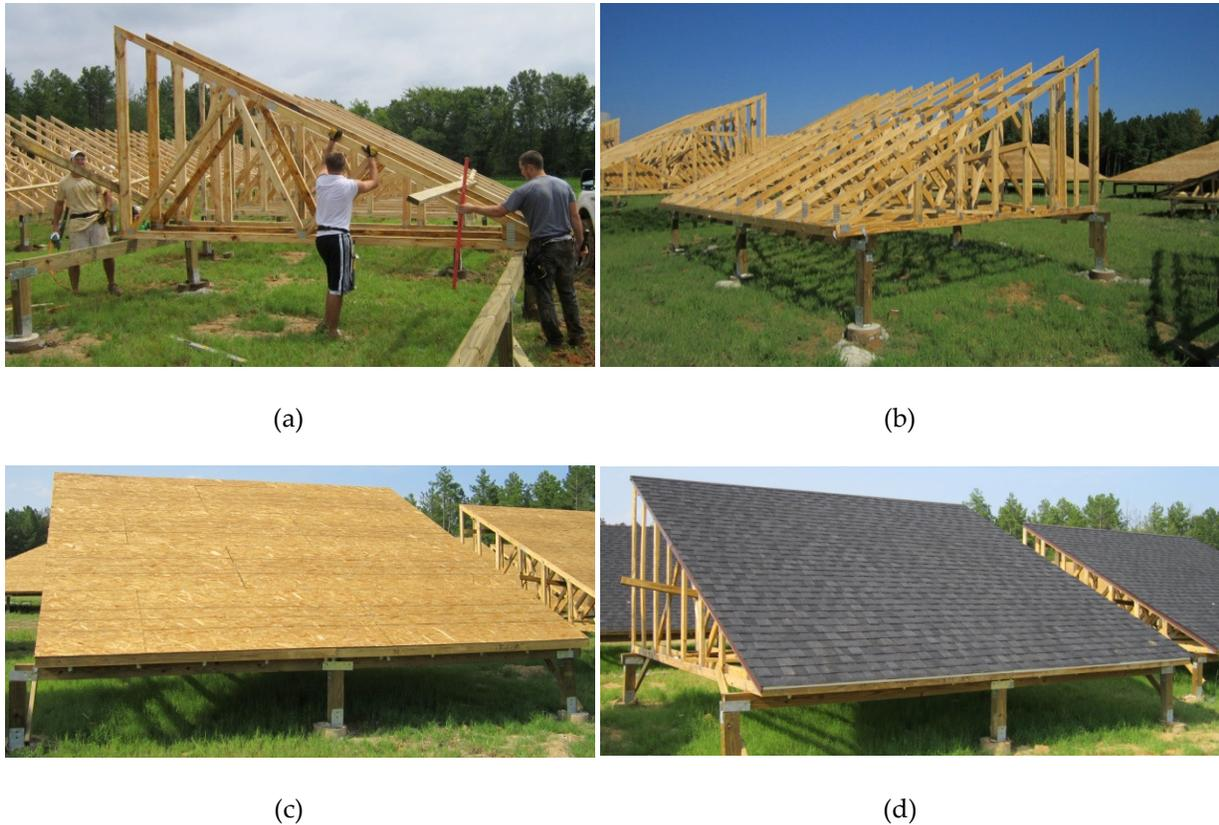
**Fig. 99. (a) - (c) Construction of the mono-slope gable roof sections. (d) Completed mono-slope gable roof section.**
