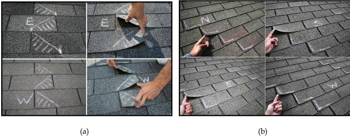
**Fig. 34. Patterns of partially unsealed asphalt shingles reported in Marshall et al. (2010). (© American Meteorological Society. Used with permission).**
